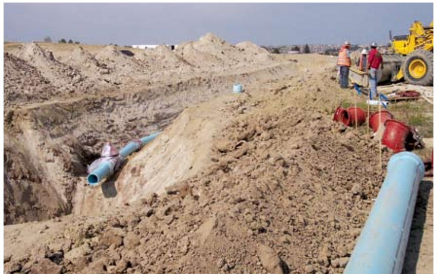
American Infrastructure puts in water, sewer and storm sewer pipelines. Here, crews are laying pipe at a single-family development in Parker, Colo.
