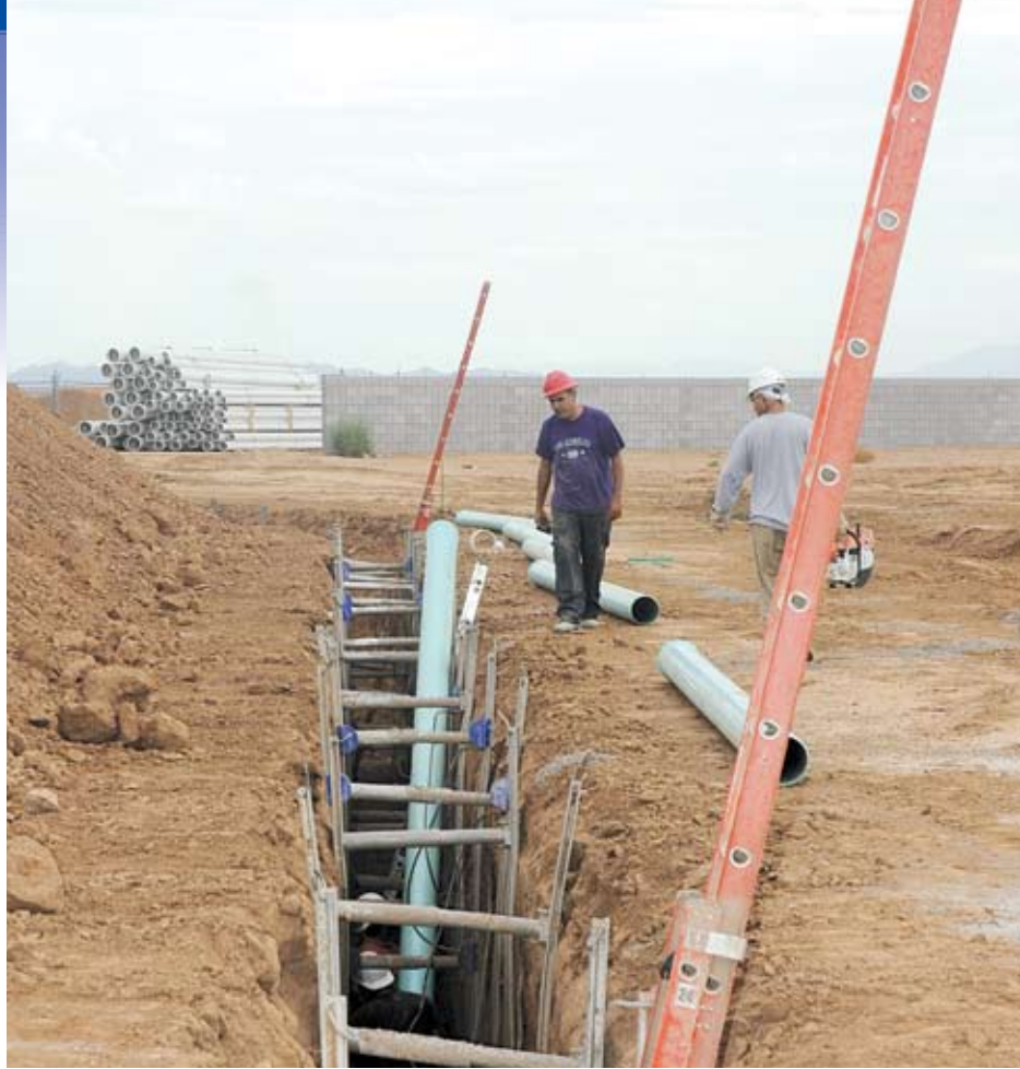
Underground contractors know good practices in trench safety are extremely important, including trench shields or boxes for deep excavations, ladders for egress at proper intervals and hard hats and other safety gear to keep workers protected from potential falling objects.
