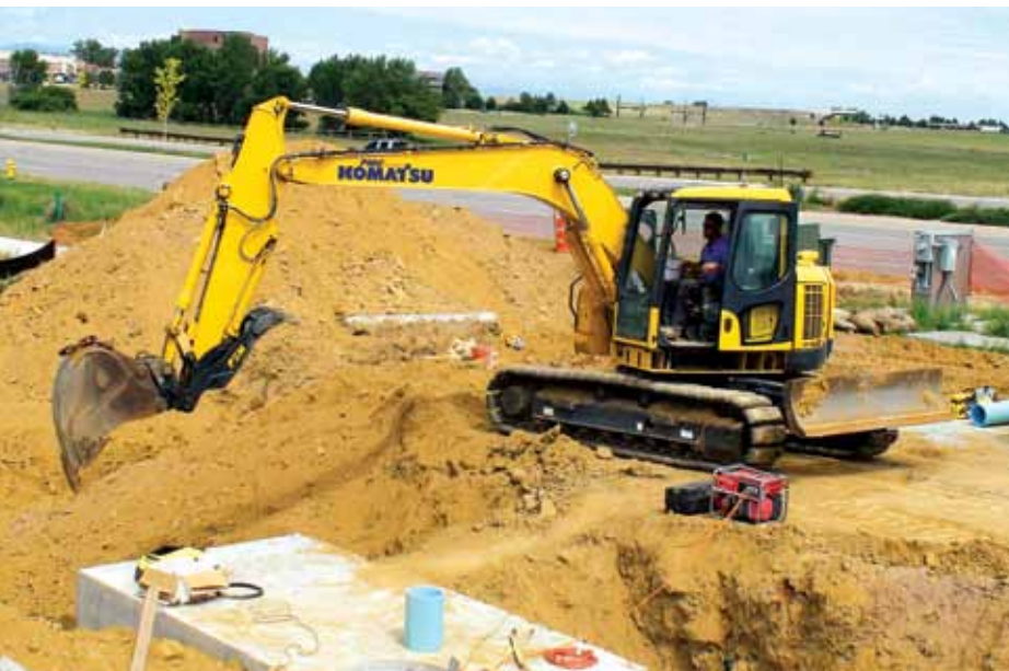
Chris Hoyt uses 53 Corporation's Komatsu PC138 tight-tail-swing excavator to install a bypass line, vaults and manholes at a job for the Arapahoe County Waste Water Authority near Centennial, Colo.
