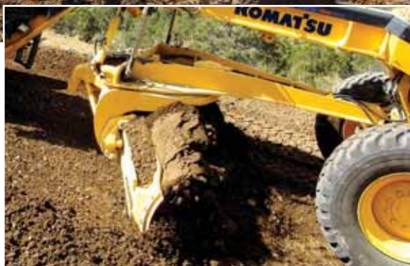
An operator for Sam Sisneros Operations uses a Komatsu GD655 motor grader to repair a road in a Trinidad, Colorado, gas field.
