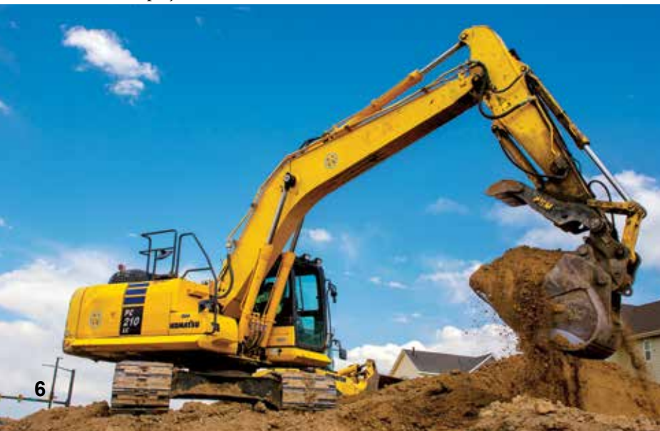
An operator digs and loads dirt with a Komatsu PC210LC excavator on a Naranjo Civil Constructors project in the Denver metro area.
